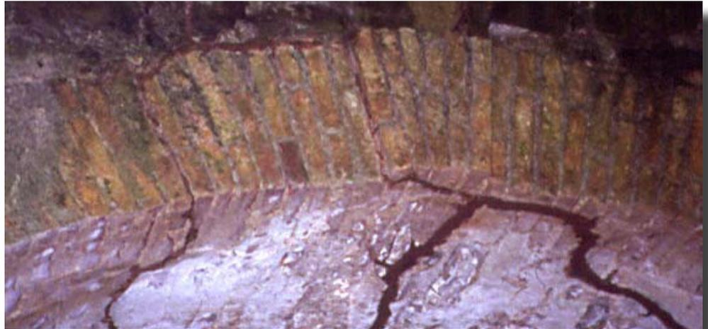
*P 3.2.8.1 The arch are built in Flensburg Stones and the arch is closed with projected key-stones.*
